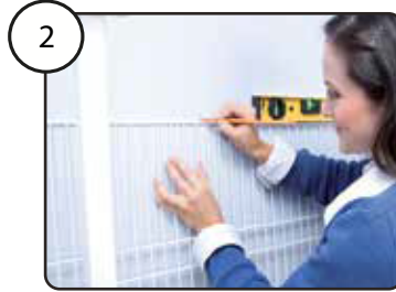
2 Nivele y marque cada 30 cm aprox. iniciando a 3 cm de la esquina. Level shelves and mark holes where the "wall clips" will be installed (The holes must be at least 12" apart).
