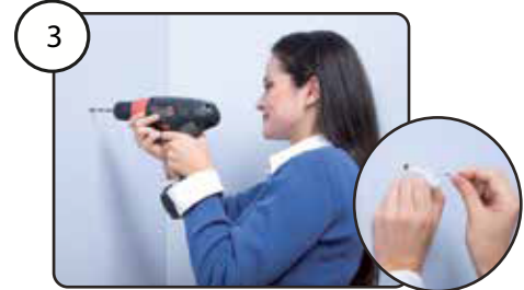
3 Perfore la pared con broca para muro de 1/4". Introduzca un "chazo J" y colóquelo un "clavo roscado". Drill each hole in the wall with a 1/4" drill bit. Insert a "wall clip" and then the "screw pin".
