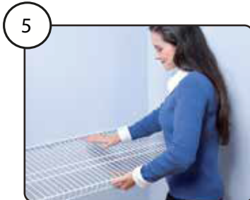
5 Instale los estantes, haciendo presión sobre los "chazos J". Set the back of the shelving into the "wall clips" and press down slowly until it locks in place.
