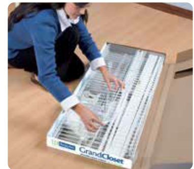
7 Haga sánduche con los "escudos", nivele y perfore el paral con la broca de 1/8", para metal y fije con tornillo. Snap in place the shelf's front between "joiner plates" attach. Use the "joiner plates" hole as a guide and insert the screw. Once the shelf is leveled, drilling a 1/8" hole into the pole.
